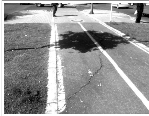
Figura 12. Fisura en diagonal causada por expansión de Subrasante Figure 12. Crossover cracking caused by sub-grade line expansion
