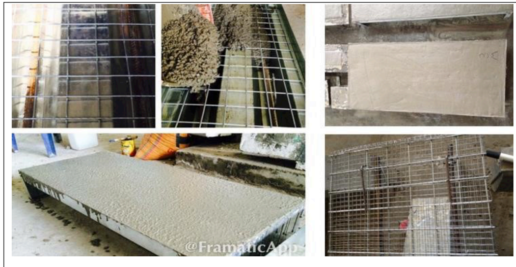
Figure 3. Cast of SCC and FER ribbed panels
