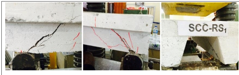
Figure 9. Web shear crack mode failure in ribs
